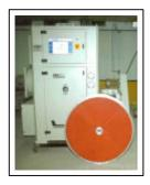
The fresh air is either precooled partially and then passed through a rotary desiccant dehumidifier, where the moisture content is reduced to the desired level. This air is passed over a heat exchanger coil fed with a cooling tower
